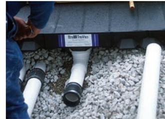
All Center and Side Track Pans are molded with pipe fitting locators at their lowest point. Below-grade piping can be installed to channel large spills to oil/water separators, holding ponds, etc.
