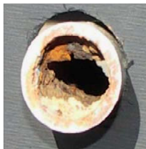
Untreated Control Pipe
