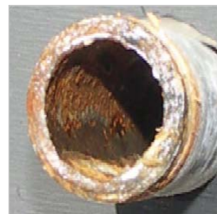
Pipe After RE-Ox Treatment
