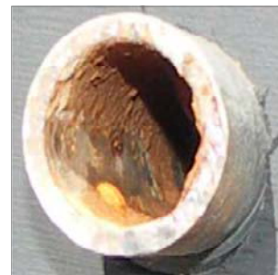
Pipe After RE-Ox Treatment
