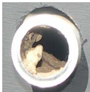
Untreated Control Pipe
