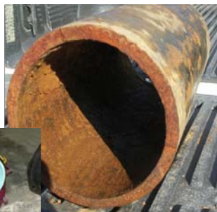
8" Pipe After RE-Ox Treatment
